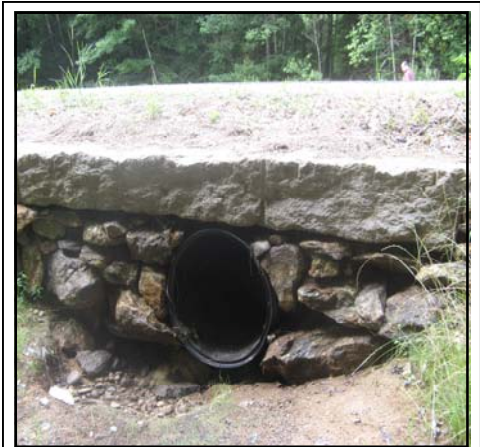
The upsized culvert on Quaker Road is stabilized with New Hampshire granite. Photo by Darby Duffin.
