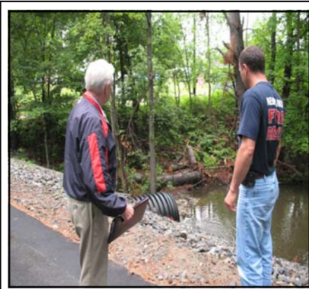
Rick Malasky (right) shows FEMA mitigation officer George Brosky (left) the larger culvert that was installed on Langs Lane in 2006. Photo by Bridget Weber, FEMA.
